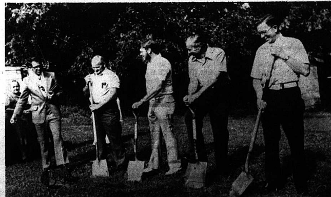
Ground Breaking Ceremonies were held Saturday afternoon at the Union Baptist Church at Red Hill. Shows above are members of the building committee as they turn the first earth for the new structure which will be located beside the present church. In the photo are, from left: Steve Day, pastor; Charlie French, Reuben Hammonds, Preston Tankersley and Arnie Taylor. [See other photos inside.]
