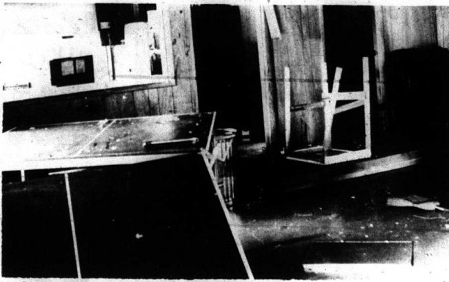
The dining area of the main building at the Kentucky Christian Camp suffered heavily from vandals last Thursday or Friday night. All wooden furniture was busted up, paneling was ripped from
