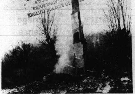
The home of Mr. and Mrs. Robert Cromer at Pine Hill was completely destroyed by fire early Saturday morning. Mr. Cromer, who is Rockcastle County's Property Valuation Administrator, said he awakened about 4:30 a.m. and realized the house was filled with smoke. He and his wife were unable to save anything, barely escaping in time themselves. The seven-room home was leveled and, it is believed the fire began around the furnace venting the furnace.
