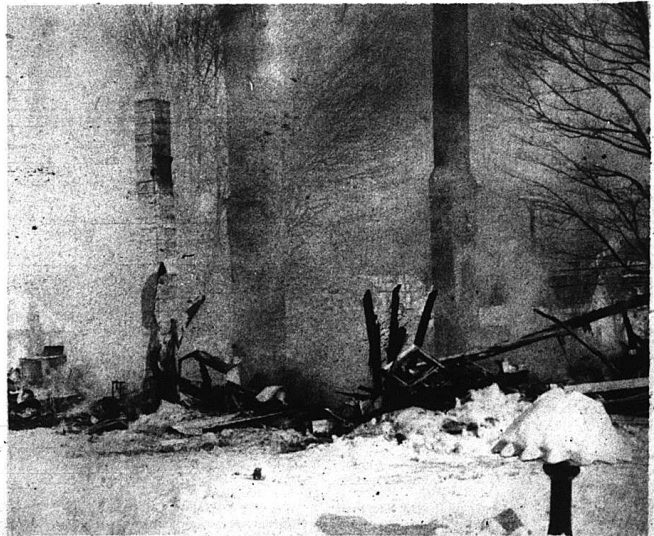
The home of Mr. and Mrs. Ray Barrier of Livingston was completely destroyed by fire Sunday night. Fire fighters from Brodhead, East Bernstadt, London and Mt. Vernon managed to
