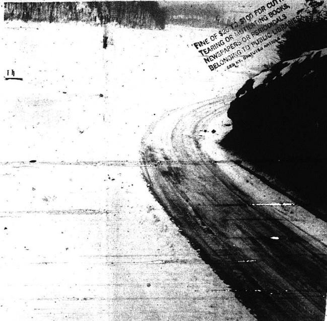
Mt. Vernon Mayor Roland Mullins has recently contacted the state Department of Highways seeking help in erecting guard rails on the more hazardous curves at Lake Linville. Within the past year two cars have slid off the road and into the water. No one has been seriously injured yet and Mayor Mullins hopes that guard rails at places such as the one above will prevent that from happening. The photo was taken near the first curve on the lake road near Interstate 75.
