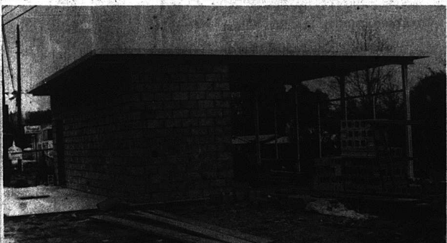
A new 8000 sq. ft. Wash is presently under construction on Richmond Street in Mt. Vernon. The new business, owned
