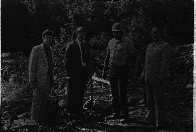
It's not much yet, but soon this spot will hold a Burger Queen. Wayne Reid, franchise owner, holds the shovel at the ground-breaking with contractor John Stephenson (wearing hat). With them (from left) are Bill James and E.H. Hamon of The Bank of Mt. Vernon, which is handling the project's financing.
