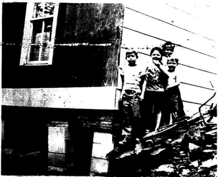
The Sturgill children in front of their house, which is only partly finished with new siding installed by the Weatherization Office.
