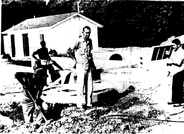
Dewey McClure, Homer Tolle, Boyd Everole and Aaron Walters built this $434,000 sewer plant for the City of Livingston. It should be operational by the end of the month.
