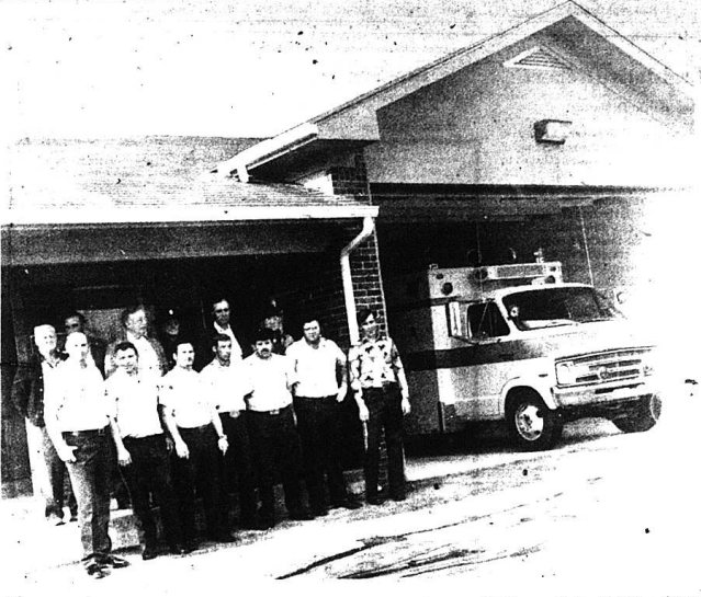
The Rockcastle County Ambulance Service moved into its new quarters, adjacent to the Rockcastle County Hospital, Monday morning and members of the Fiscal Court were on hand for the occasion. Shown in the above photo are several of the drivers. From left: Stanley Mullins, Delmo McClure, Hershall Callahan.
