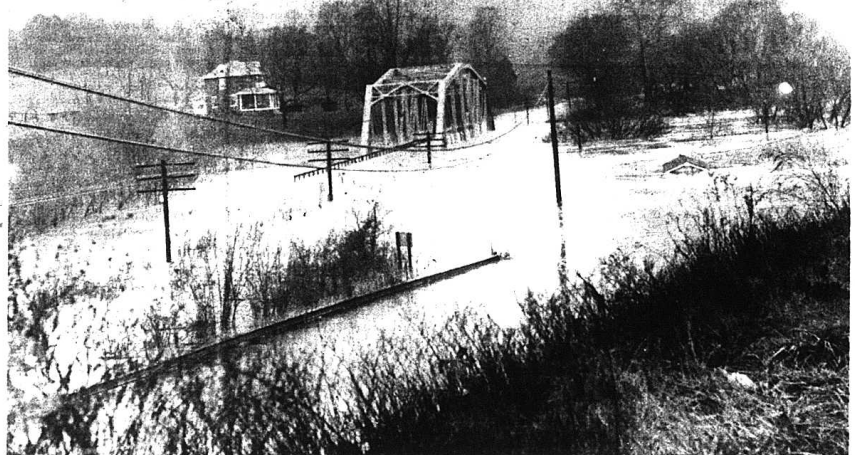
The City of Livingston's new $433,000 sewer plant, which was completed in late summer was covered by flood
