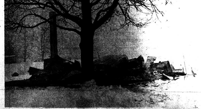
A house, owned by Beale Brock, in Seafield Court burned down last night. The house was owned by Beale Brock and his children had rented the house but were not home at the time of the fire. Mr. Vernon was called to a fire about 3 a.m. Saturday morning at the home of Mr. and Mrs. Jesse Tucker in Fairground Hill. Fire Chief John Cox said that Mrs. Tucker was not home and her children were not home at the time of the fire. The house was estimated to be worth between $500 and $1000, according to Chief Cox.
