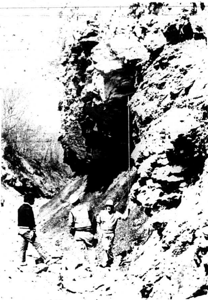
They are not mountain climbers, but a crew from the State Department of Highways, measuring the rock overhang on U.S. 25. Ronald Rice, the man in charge, said that some of the rock would be removed between 1978-80.
