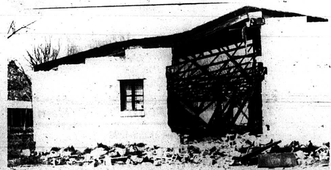
The slaking rink at the fairgrounds is partly demolished. The job should be finished within a week
