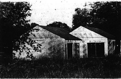
A community center for senior citizens and the handicapped, is shaping up at the Brodhead Fairgrounds. This picture was taken this week and shows that the building is almost completed. It will be used to house 4-H Exhibits at the Fair this August.
