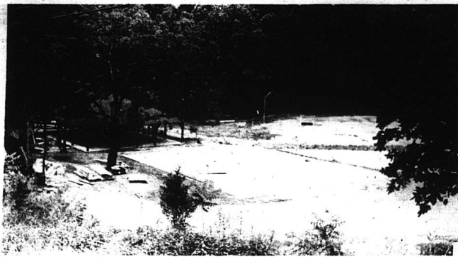
A recreation center has been built on the old Parsons Property near Renfro Valley and is open to the public July 7. On the right is a pavilion under which table
