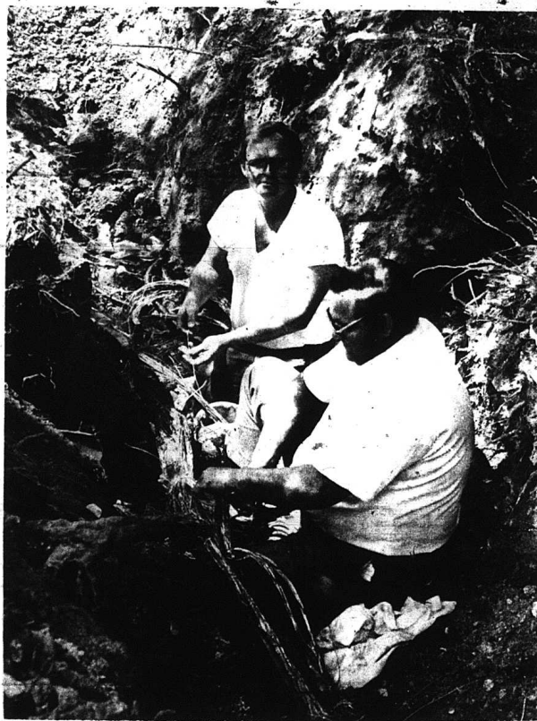
Ron Handley, left, and Bill Dewey, cable splicers for Continental Telephone Co., were busy Monday afternoon repairing an underground cable behind City Hall, which
