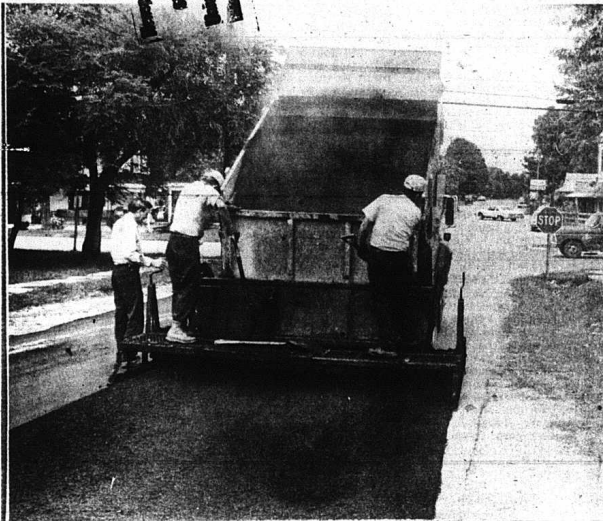
City employees are shown in the above photo blacktopping on Williams Street. Several streets in town received complete resurfacing while all the potholes were patched in preparation for winter weather.
