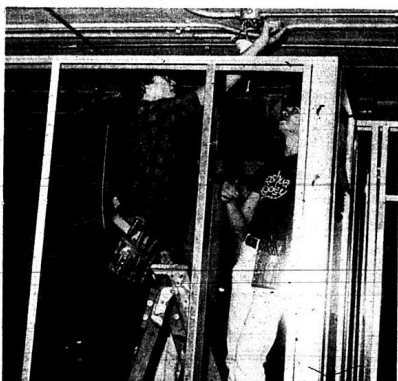
Members of the Harry Sparks Vocational School Electricity Class are donating their time to the hospital by wiring the addition which will house the new surgery department and the offices of Dr. Yip and Thomsen. Altogether, 18 high school students and 8 adult students, along with their instructor, Jack B. Dalley, are working on the project. In the above photo, Scott Stewart, left, and Mike Stewart are shown installing a ceiling fixture.
