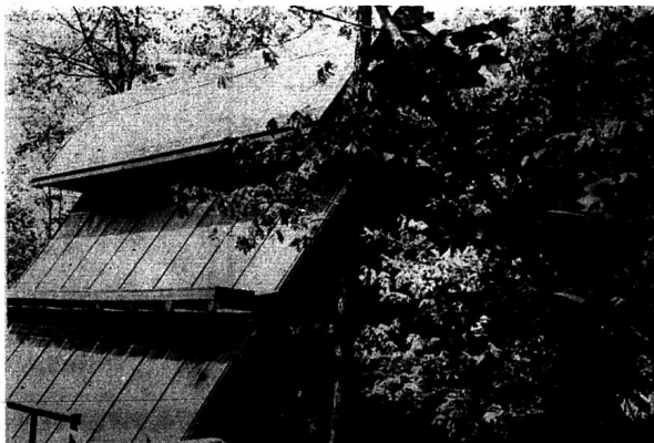
A view showing the back and southern exposure of the model solar home being built below Livingston.
