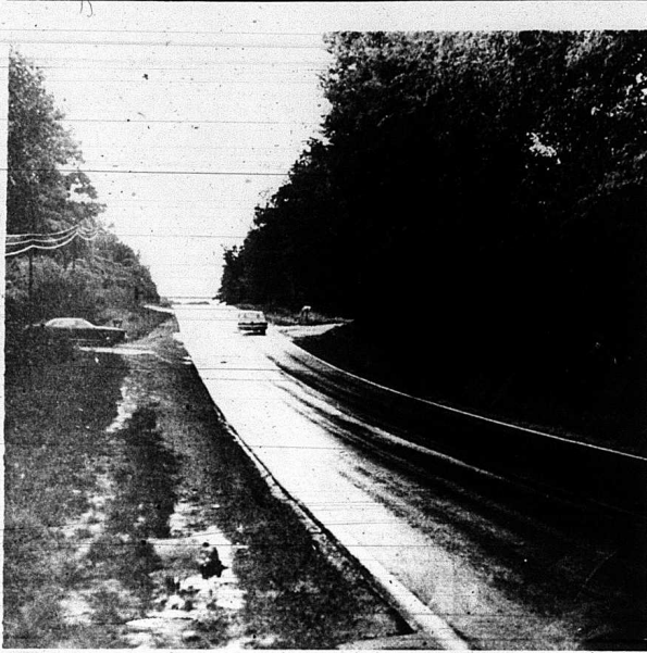
A $570,238 contract has been awarded to Elmo Greer Associates, G&G Kentucky Construction Co. and G&C Coal and Energy Corporation, all of London, in a tri-venture to construct 0.8 miles of U.S. 150, Mt. Vernon-Broadhead Road, from about 240 feet west of Ky. 461, extending westerly. The
