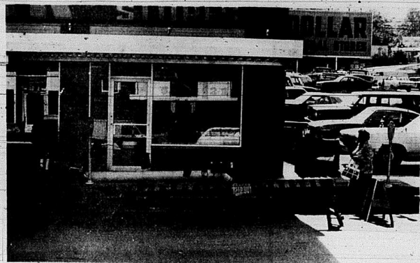
A leak in gasoline storage tanks at a station, belonging to Wayne Bullock on 150, caused gasoline to collect in caves under buildings located on Main Street. The situation became potentially explosive last week. Fuel was removed in the General Dollar Store and state and
