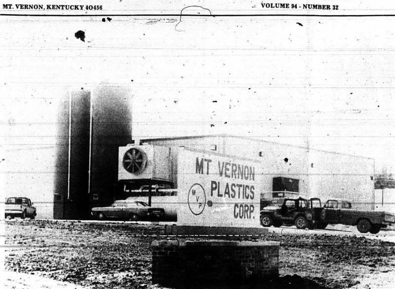
Mt. Vernon Plastic Corporation is scheduled to begin production next week. The newest addition to the Rockcastle Industrial Park is a newly formed company in which four men from
