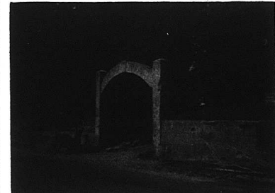
In 1970 the Rockcastle County Jaycees hired workers to rebuild the crumbling concrete wall at Elmwood Cemetery and remove the arch which had been erected in 1921.
