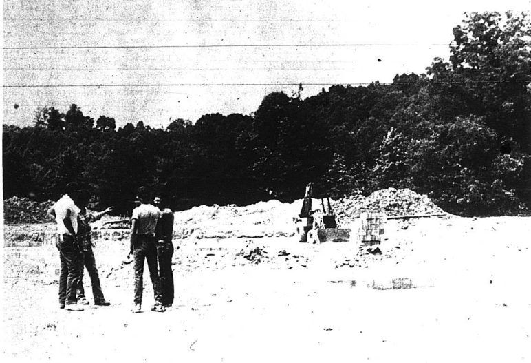
Construction began five weeks ago on a 70 unit housing project at Brodhead near the Fairgrounds. The project will include 13 apartment buildings plus an office and laundry building. Projected completion date is June 25, 1983, according to Jim Houston, superintendent of construction. From left, are Houston (of Morrow, Ohio,
