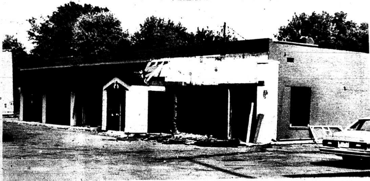
Rockcastle County's new health department will be built on the above site of the old Dinner Bell Building. Demolition work is being done by Clarence Hasty of Mt. Vernon who submitted the low bid of $999. Health Board Chairman Attorney Jerry Cox said Wed-
