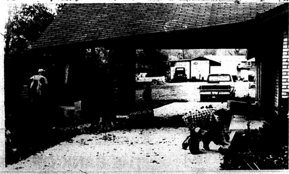
Gary Kerr, a member of the Jehovah Witness Church on Poplar Street in Mt. Vernon, is shown as he cuts off a support to put under the front corner of the carport on the church. Two of the carport's three brick supports were knocked out by Glenn Pitman, 45, of Mt. Vernon, who
