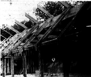
The dining hall under construction at cleftRock will seat 40 comfortably. Materials for the building are expected to cost $50,000. Labor is volunteer.
