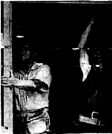
The Rockcastle County Health Department Building is now under construction and has been for several months. No date has been set for the completion of the project. In the above photo, Jim Arnold, left and Kenneth DeWitt are shown as they work on one of the door facings in the building. Built-Wel Development Corporation has the contract on the building.
