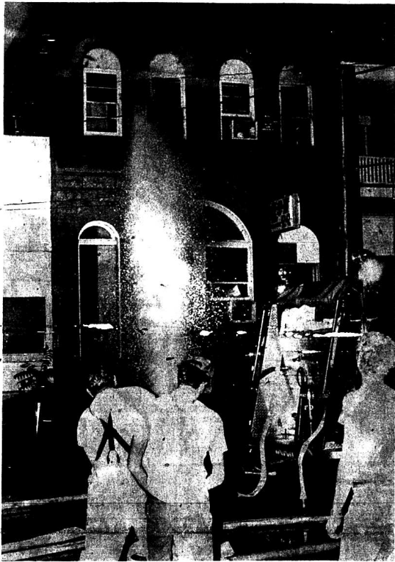
Mt. Vernon firemen battled a fire in a Main Street building Monday morning from about 1:45 to 7 a.m. The fire, which apparently started from overloaded wiring in a central area upstairs, completely gutted the building which also housed the pool hall. The building was owned by
