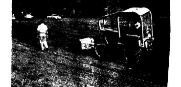
An 850 ft. diversion channel is shown being constructed recently on the Paul Abney farm at Wildcat. The diversion channel, built to protect a tobacco field below, was shaped completely with a bulldozer and has been seeded with fescue.
