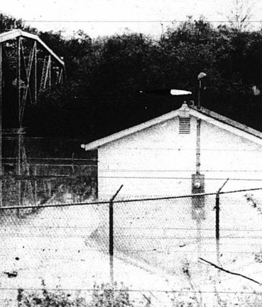
The Rockcastle River crested at about the level shown in the above photo taken about 7:30 Monday night. In the foreground of the photo is the Livingston Sewer Plant which had to be made inoperative Monday afternoon because of rising flood waters. Railroad officials didn't take a chance on the railroad bridge, shown in the background. When rising flood waters threatened the bridge, several railroad cars were pulled across it to help "hold it down."
