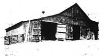
This is a 48x65 combination stock and tobacco barn including sheds with metal roof, still in good usable condition.
