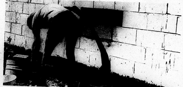
Another break-in... Franklin's Variety store in the West Gate center in Mt. Vernon was robbed last Monday night. A workman is shown in the above photo fixing the hole in the wall.
