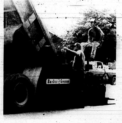
Getting ready for School . . . Johnny Newland of Newland Construction Company of Berea is shown above giving instructions to one of his employees. Newland was present Tuesday blacktopping in the Mt. Vernon Grade School parking as the county systems gets wound up for school to open on August 16th. Enrollment for students will be on August 17th.
