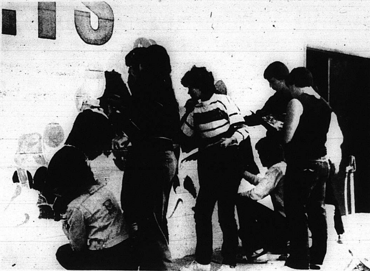
RCHS Art students and Lawrence Bullock are shown painting the art work on the new football dressing rooms at the high school. Material for the two buildings were furnished by the school board and the majority of the labor for construction was
