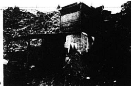
Pictured above is 80 ton unloading hopper and crusher equipment.
