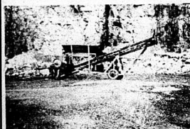
Portable Crusher pictured above is a large crusher w/6 cyl. Niassan Diesel Engine.
