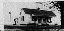
House - 1 Acre Lot - Bonnie Ridge - House has 3 bedrooms, living room, kitchen, dining room and bath. Also built-in back porch, city water, level lot. All for $19,500. 115.
