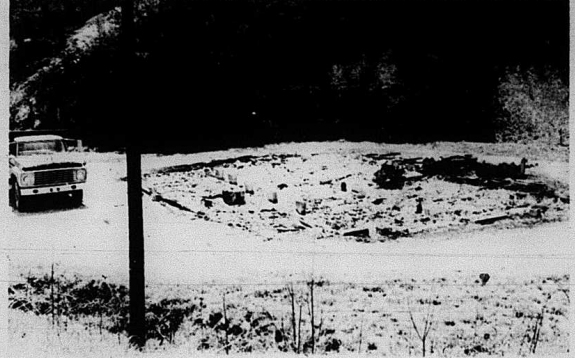
Only ashes remain of what was once the Calloway Holiness Church that burned last week. Livingston Fire Chief Jerry Mink said Livingston city police reported the fire and, when firemen arrived at the scene, the building was already engulfed in flames.
