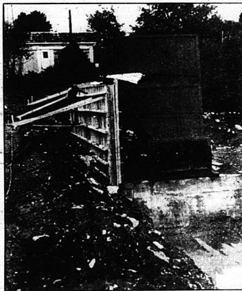
A garbage compactor is under construction south of I-75 interchange at Burr that will be used by Bee Garbage Transfer Systems of Mt. Vernon to press collected commercial garbage in Mt. Vernon. Johnny Eaton, owner of Bee, said the compactor will be completed in about a month. Eaton said no liquid will escape from the concrete holding basin.
