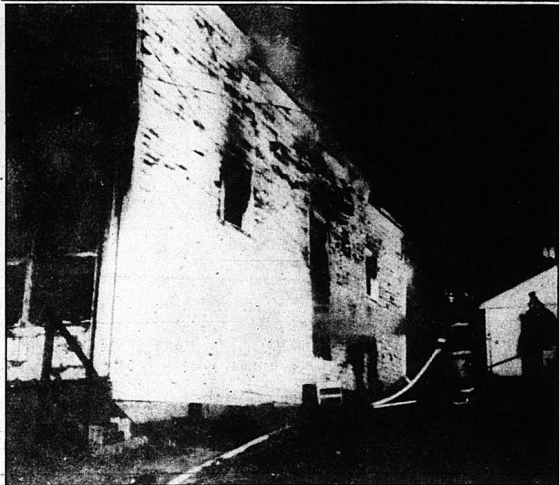
ONLY CHARRED INTERIOR REMAINS OF LOCAL CHURCH
