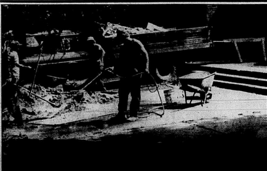
Work is continuing on remodeling at the Rockcastle County Jail. The expanded facility is expected to be completed in late November. Contract for the facility was awarded to McKnight and Associates of London. Included in the remodeled jail will be a drunk tank and visiting area.
