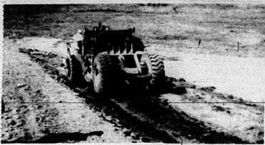
A 6-7 acre lake on the farm of Noah Poynter in the Level Green section on 461 has been dug. Mr. Poynter said the lake, which will be a pay fishing lake, will be stocked with different kinds of fish
