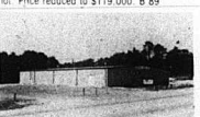
COMMERCIAL BUILDING AND LOT - South of Mt. Vernon on US 25. Building and business. Walk-out deal. Rockcastle Roller. Link. Although the building is being utilized as a skating rink, it could be adapted to most any type business. 70 x 125. Records available to qualified prospects. $185,000 B 12
