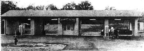
Danny McKinney recently built a four bay car wash in Brodhead.
