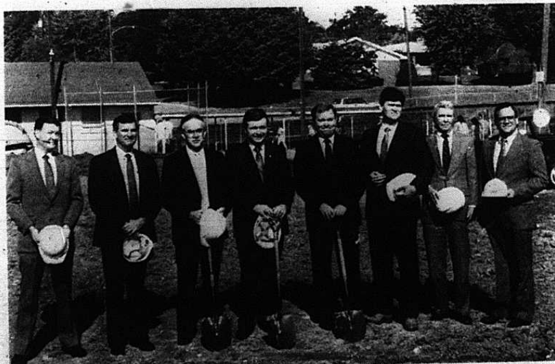
Groundbreakers at the site of the new Mt. Vernon Elementary School were, left to right, George Poynter, chairman of board of education, Dr. John Brock, State Superintendent of Public Instruction, County Superintendent Bige Towery, Jr., State Representative Danny Ford, John Hale, principal, Garlan Vanhook, architect, Fred Dupree, Jr., fiscal agent, and Stephen Branscum, general contractor.
