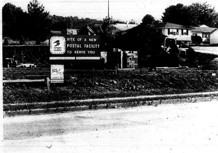
Excavation began recently for the new post office in Mt. Vernon, located at Richmond and Lewis Sts. The new facility is expected to be completed next March. The cost has been put at $329,659, and DWB Builders of Flat Lick is the general contractor. Adequate parking is expected to be one of the features of the new post office. The current office on Main St. lacks parking, both for customers and mailmen, and mail service trucks.
