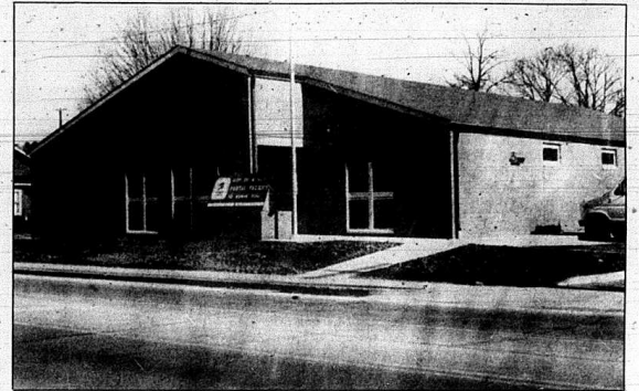
New post office at Mt. Vernon is nearing completion and is expected to be occupied by the end of February.
