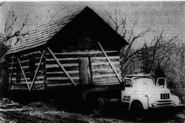
Things are "moving and shaking" at Renfro Valley these days and the original Red Bud School House was moved last week into Renfro Village.
