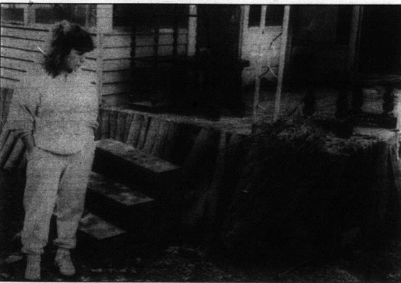
Rhonda Durham looks at debris left by the rain that flooded her trailer on the Old Conway Road at Roundstone Sunday night. The water got as high as five feet upon the trailer after Roundstone Creek flooded it's banks.
