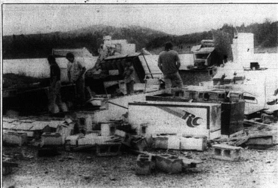
Lake Linville boat dock operator Jimmy Hale and others survey the damage to the main building at the dock. Tuesday afternoon's storm ripped the roof off the building and destroyed most of the contents.
