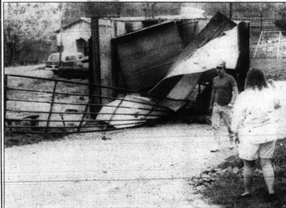
Linda McWhorter prepares to look at the damage done to a trailer that was overturned just north of Renfro Valley by the severe storm that hit the county Tuesday. McWhorter's sister, Nancy Kirby, was preparing to move into the trailer in a few days. Ironically Mrs. Kirby lost her home to a fire last week.
