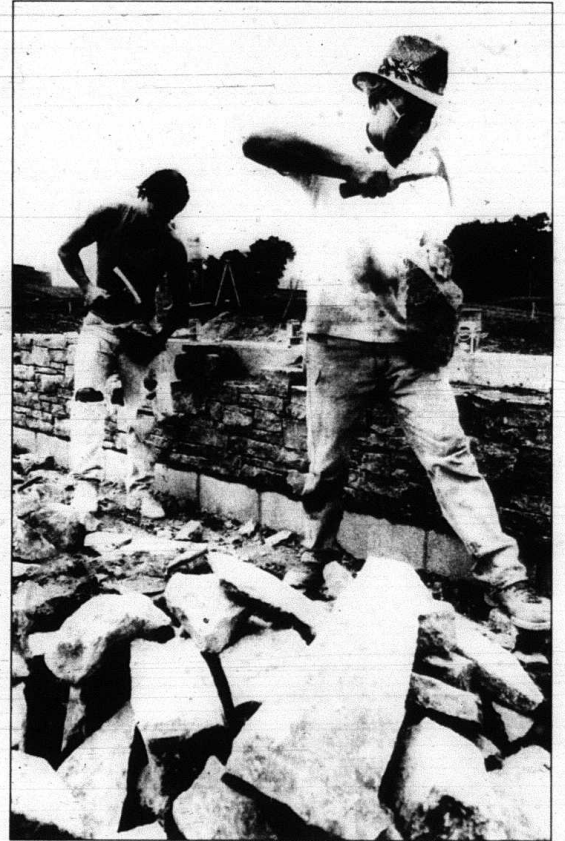
Wendell Renner and his son Tony of Orlando were busy last week chipping limestone for a wall that will run through the center of Thoroughbred Park. The photo appeared in the Lexington Herald-Leader.
